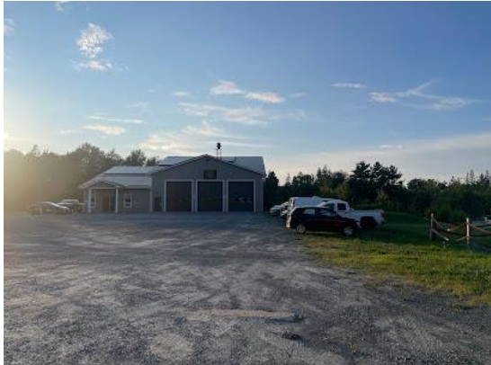
Blockhouse Fire Hall 2017, $824,000
